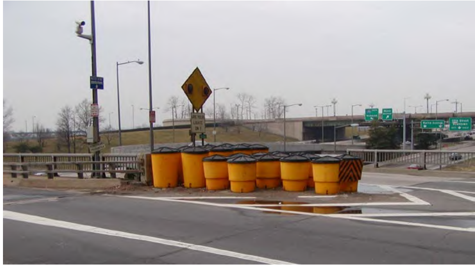
Figure 7.6.16 Impact Attenuator
