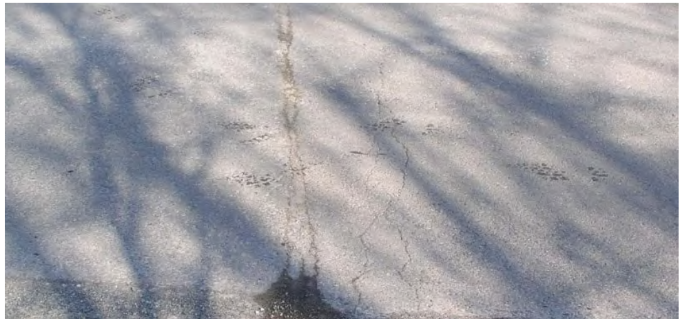
Figure 7.5.28 Asphalt Wearing Surface over an Expansion Joint
