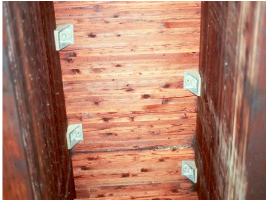
Figure 7.1.3 Glued-laminated Deck Panels Attached to Superstructure
