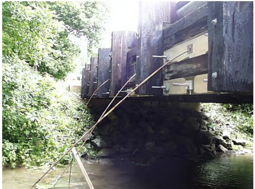
Figure 7.1.11 Broken Prestressing Anchors
