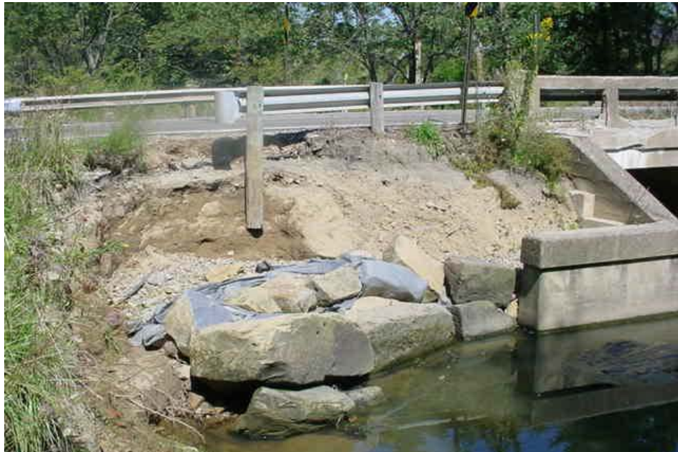
Figure 7.6.14 Erosion Reducing Post Embedment
