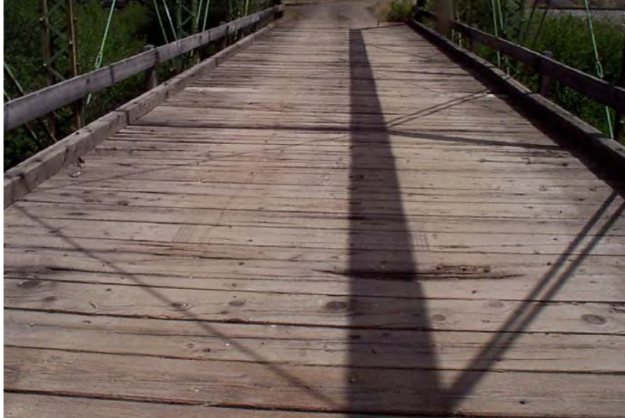
Figure 7.1.1 Plank Deck
