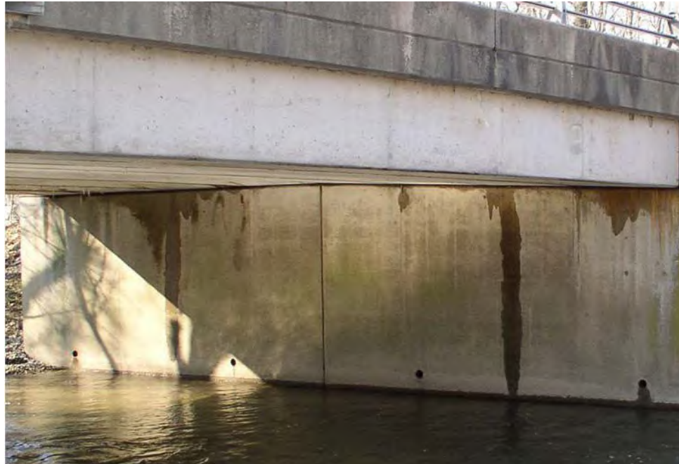
Figure 7.5.23 Weep Holes
