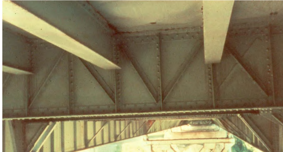
Figure 7.4.2 Underside View of Buckle Plate Deck
