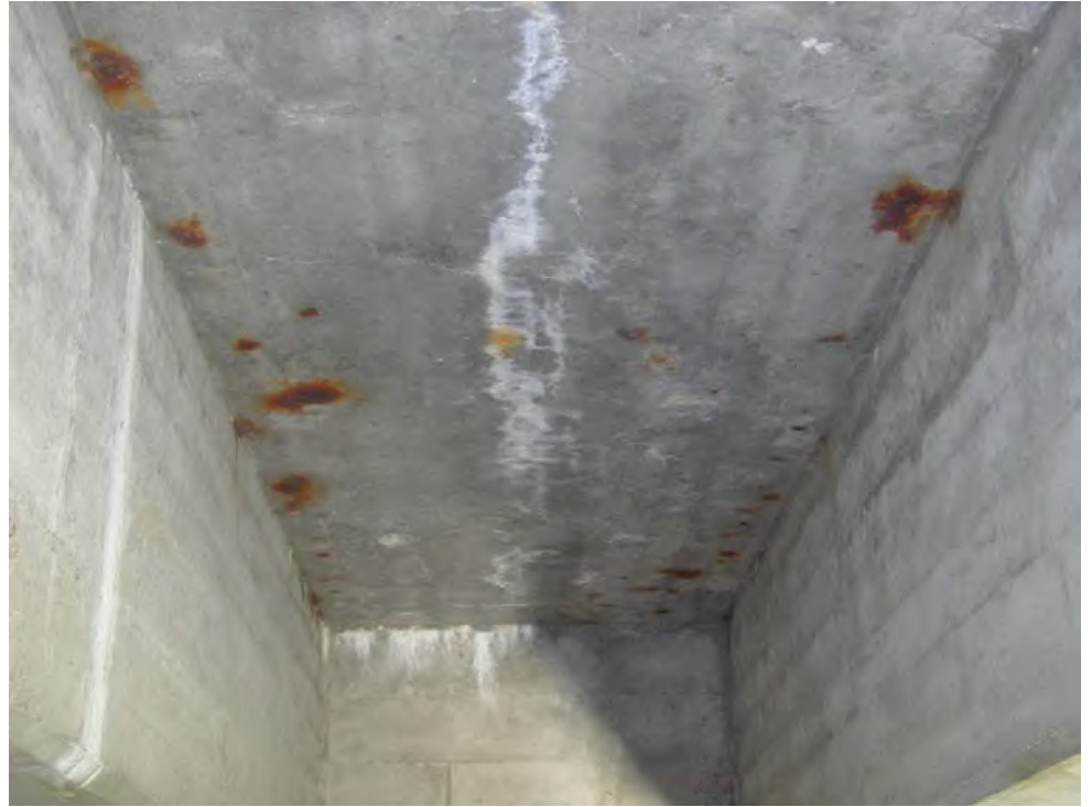
Figure 7.2.8 Underside View of Longitudinal Deck Crack
