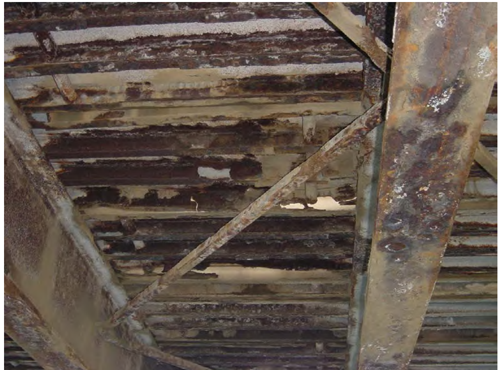
Figure 7.2.9 Deteriorated Stay-in-Place Form
