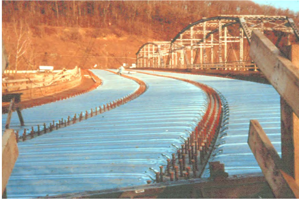
Figure 7.2.3 Shear Connectors Welded to the Top Flange of a Steel Girder for Composite Deck
