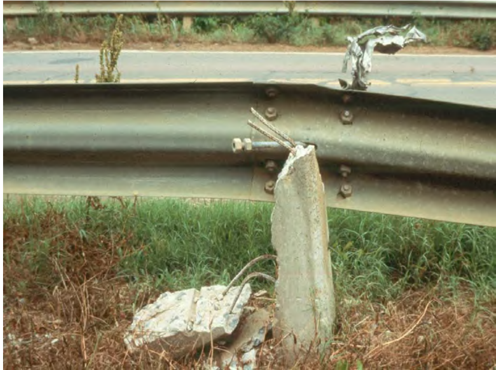
Figure 7.6.13 Approach Guardrail Collision Damage
