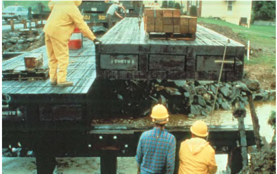
Figure 7.1.5 Structural Composite Lumber Deck Using Box Sections
