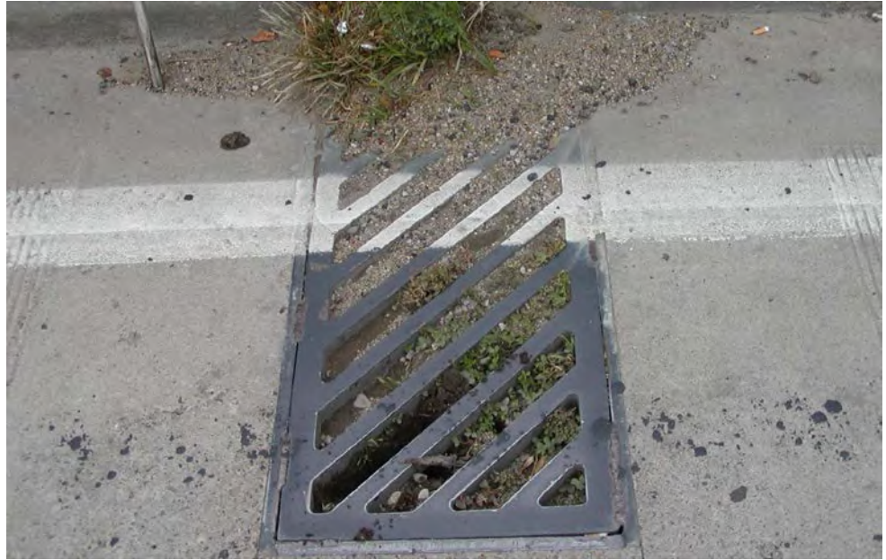
Figure 7.5.30 Clogged Scupper
