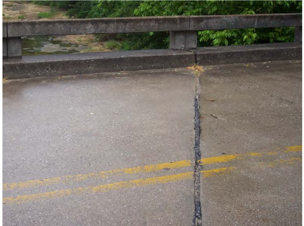
Figure 7.5.2 Pourable Joint Seal
