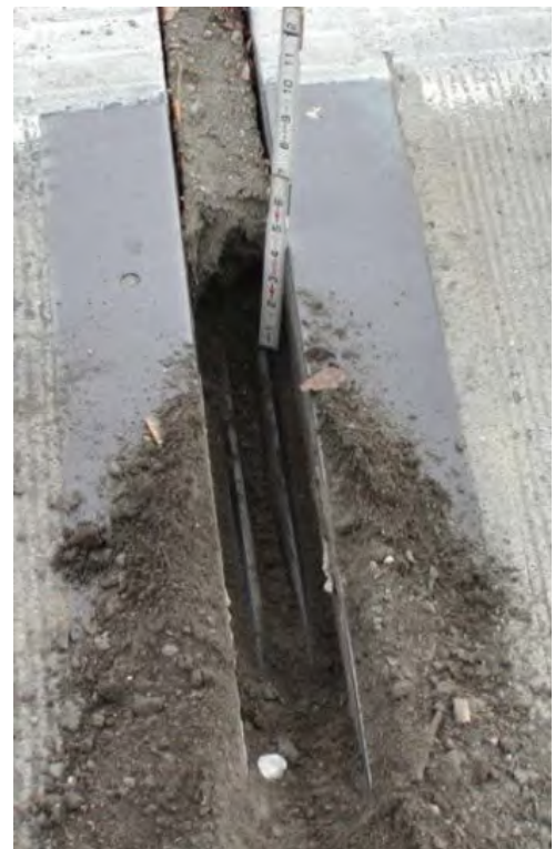
Figure 7.5.25 Dirt in a Compression Seal Joint
