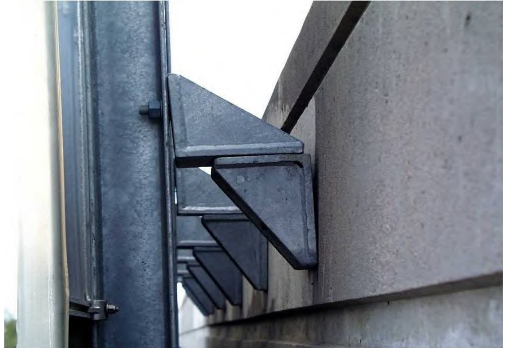
Figure 7.5.35 Sign Mount with Loose Adhesive Anchorage
