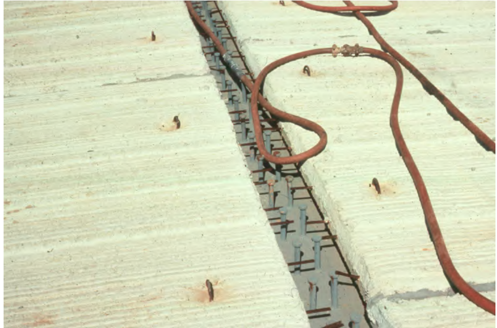
Figure 7.2.2 Precast Deck Panels with Lifting Lugs Evident and Top Beam Flange Exposed (Prior to CIP Topping)
