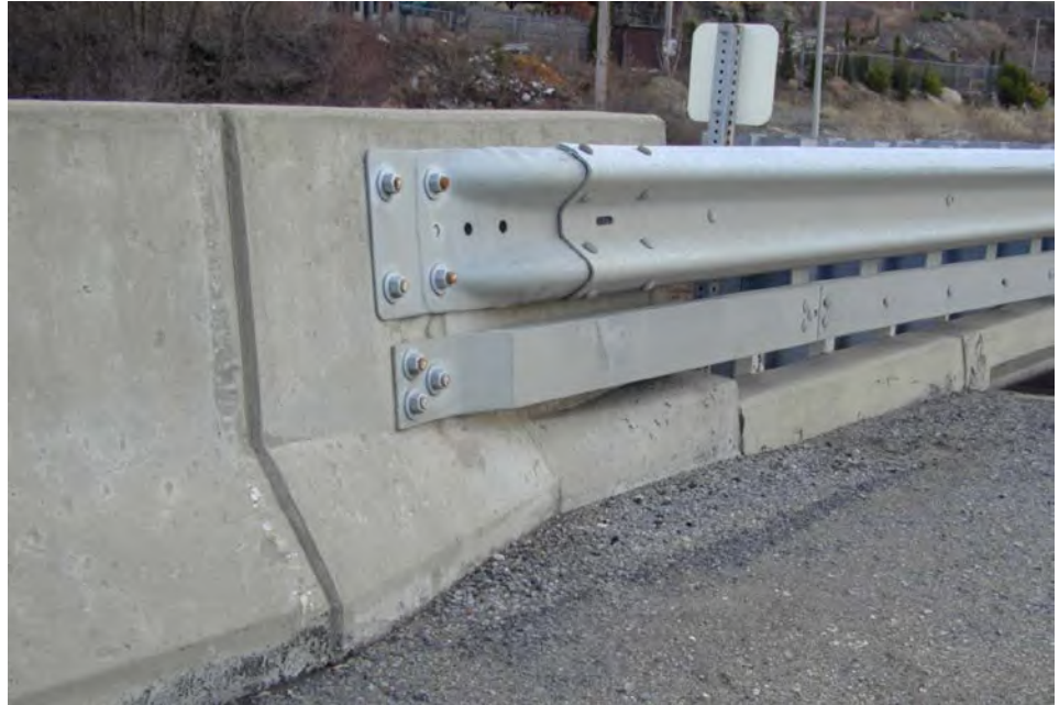
Figure 7.6.15 Proper Nesting of Guardrail at Transition
