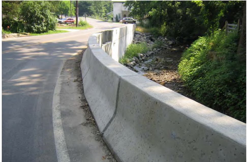
Figure 7.6.6 Acceptable Bridge Rail
