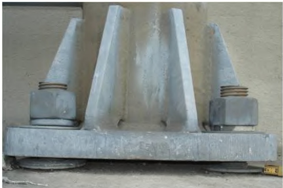
Figure 7.5.34 Sign Attachment Exhibiting Anchor Pullout
