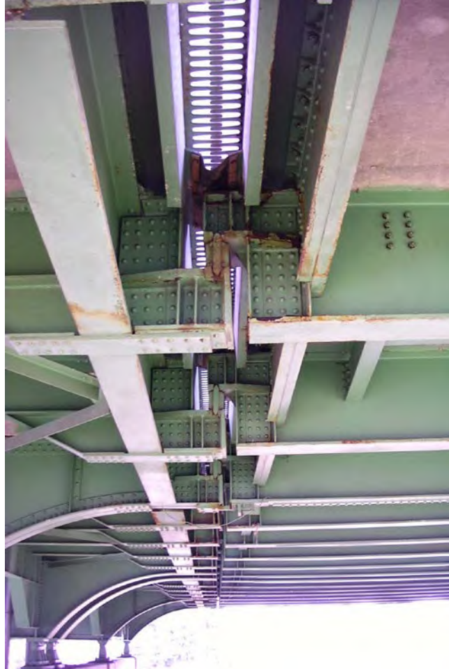
Figure 7.5.29 Support System under a Finger Plate Joint
