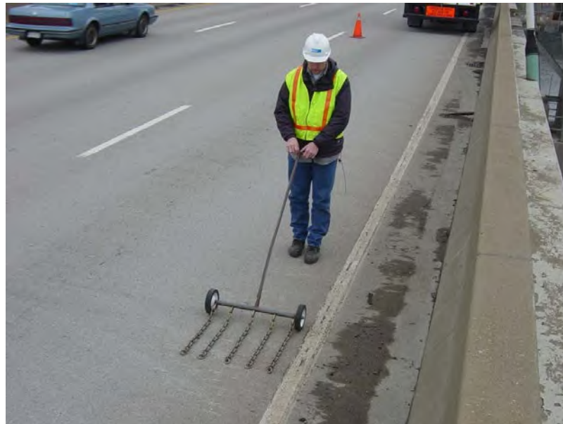
Figure 7.2.7 Sounding for Delaminated Areas of Concrete
