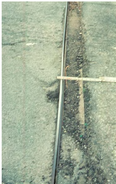
Figure 7.5.24 Debris Lodged in a Sliding Plate Joint
