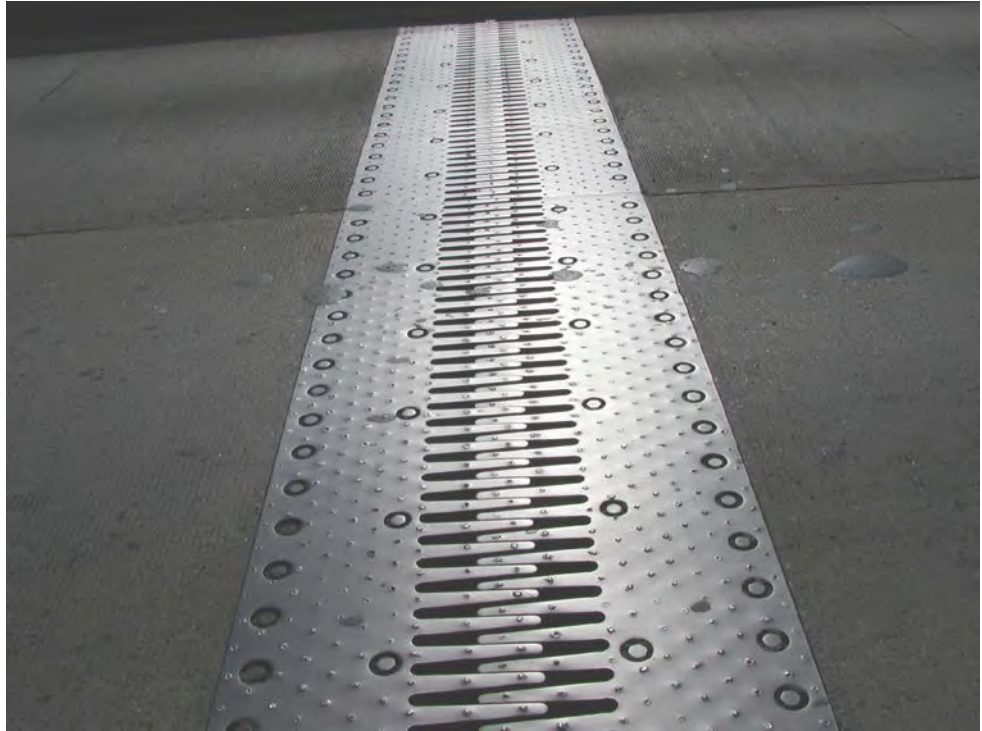
Figure 7.5.14 Finger Plate Joint
