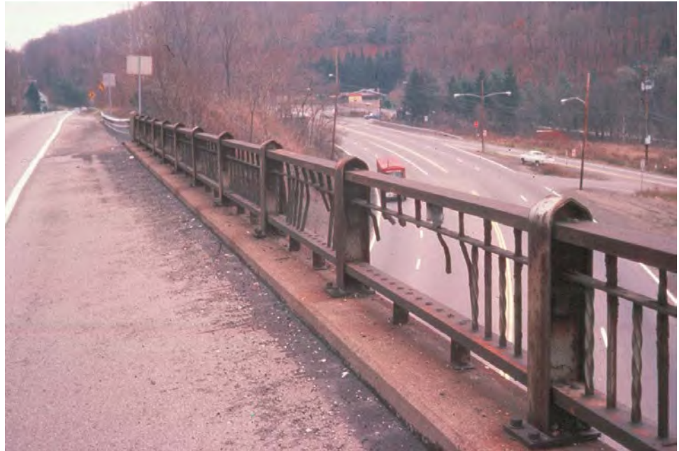
Figure 7.6.12 Deficiency Steel Post Bridge Railing
