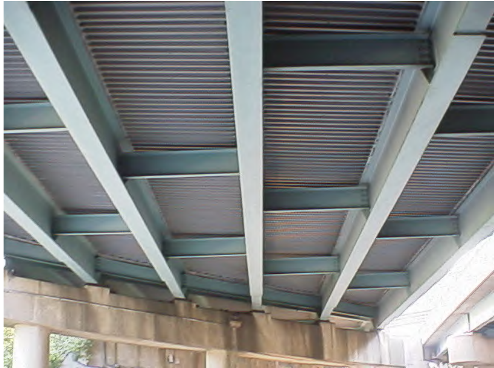
Figure 7.2.1 CIP Concrete Deck with Stay-in-Place Forms
