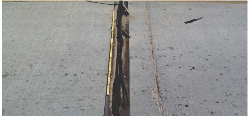
Figure 7.5.27 Failed Compression Seal
