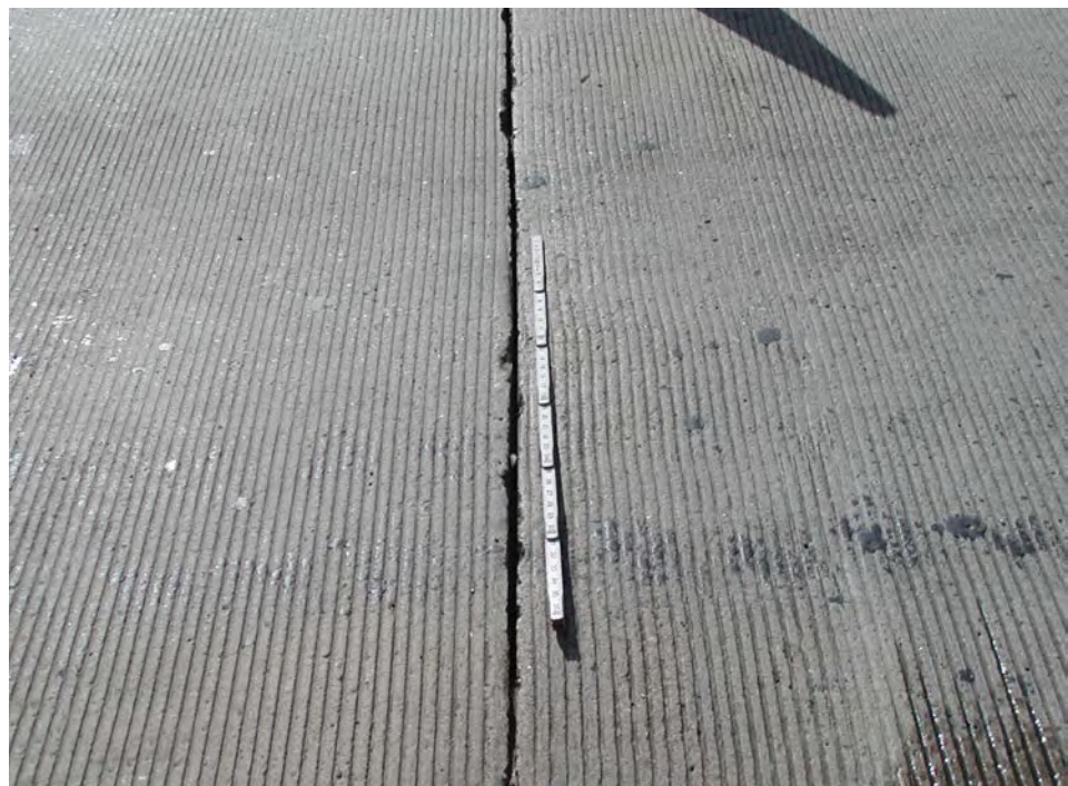
Figure 7.5.12 Open Expansion Joint
