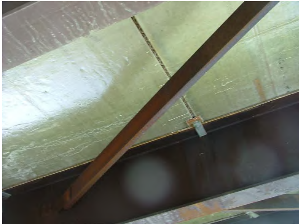
Figure 7.3.1 Fiber Reinforced Polymer (FRP) Deck
