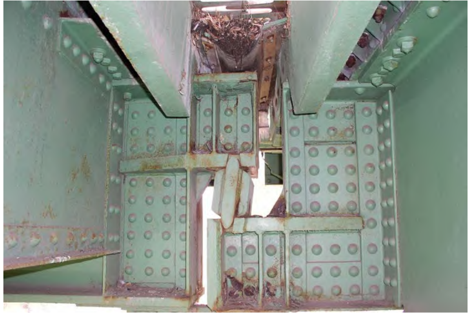
Figure 7.5.32 Drainage Trough with Debris Accumulation
