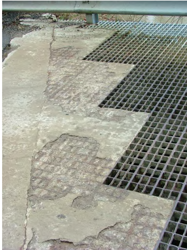
Figure 7.4.8 Filled and Un-filled Steel Grid Deck
