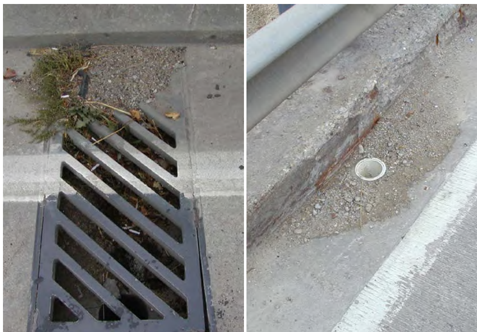
Figure 7.5.19 Bridge Deck Scupper (left) and Deck Drain (right)
