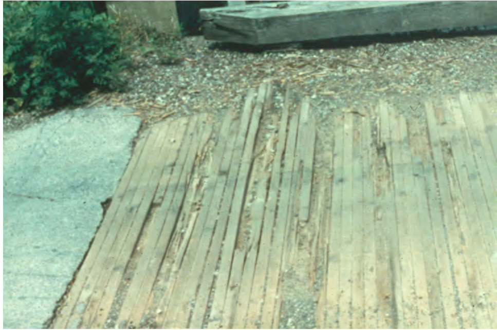
Figure 7.1.8 Wear and Weathering on a Timber Deck
