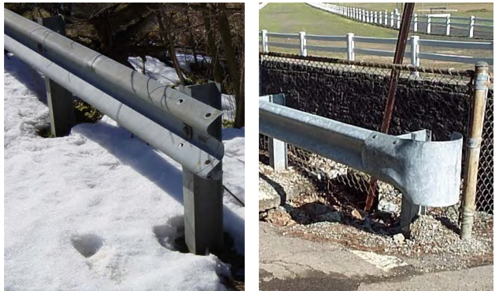
Figure 7.6.11 Unacceptable Blunt Ends
