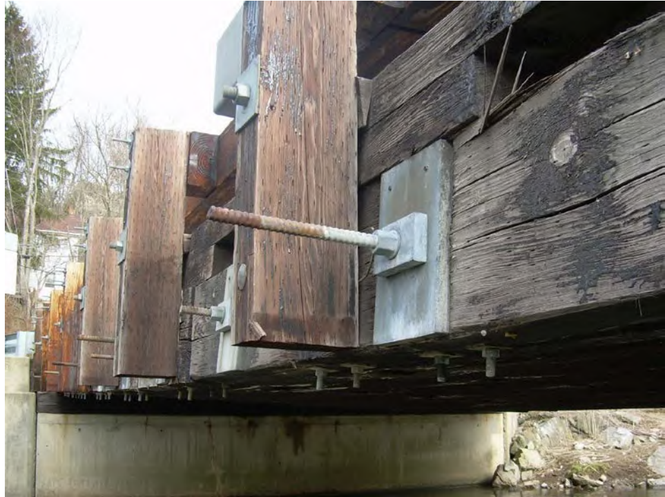
Figure 7.1.4 Stressed-laminated Deck
