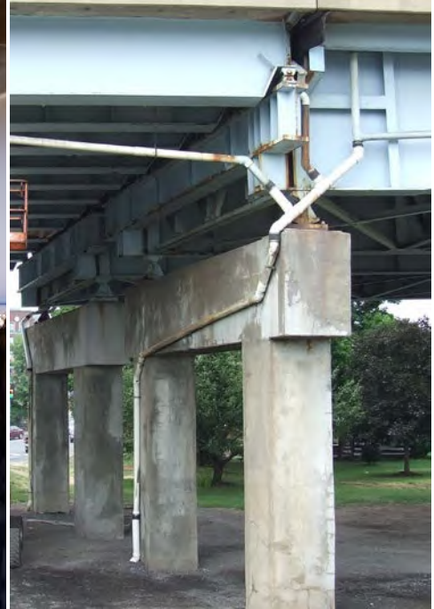
Figure 7.5.21 Downspout Pipe
