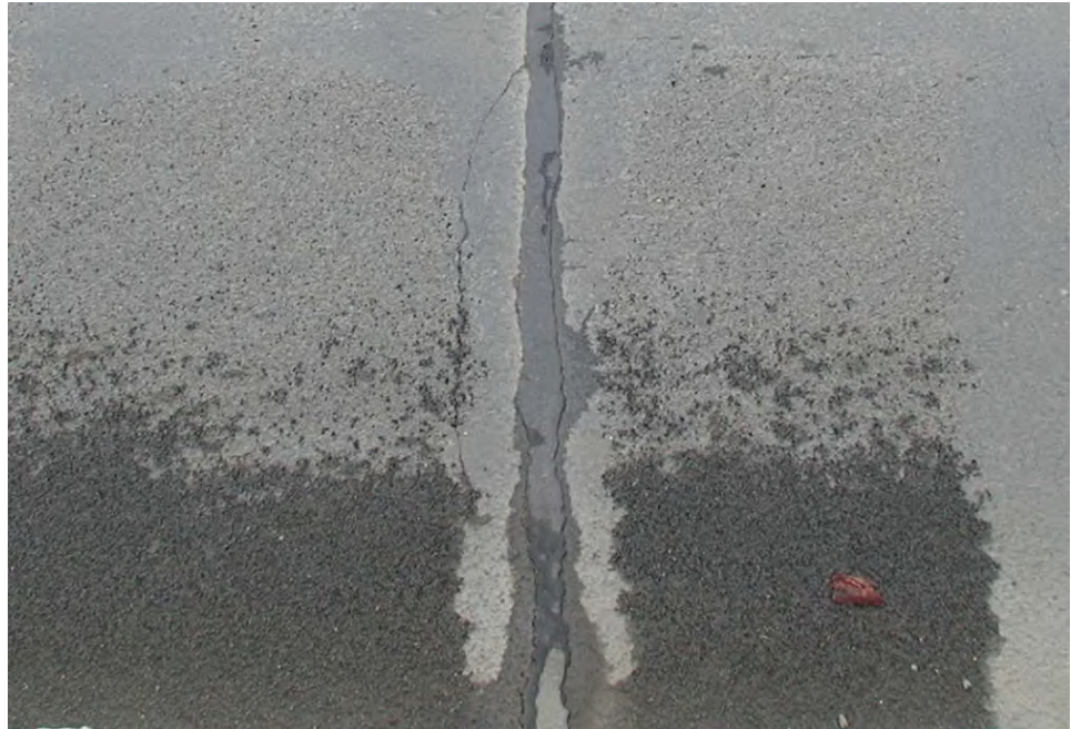
Figure 7.3.7 Deck expansion joint
